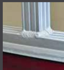
Welded then Anodized Rail Supports
